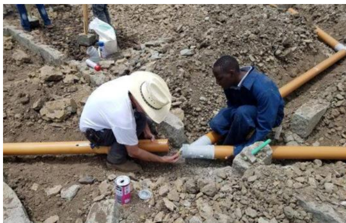
Daniel Hill demonstrates for Alex the technique of properly connecting sewer pipes in new home construction.
